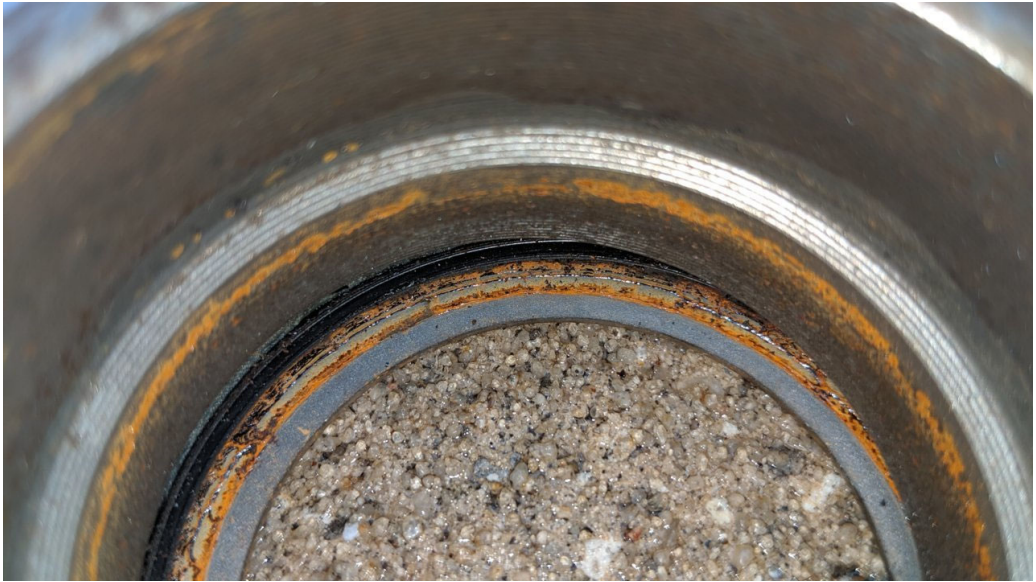
detail B properly resting against seal
